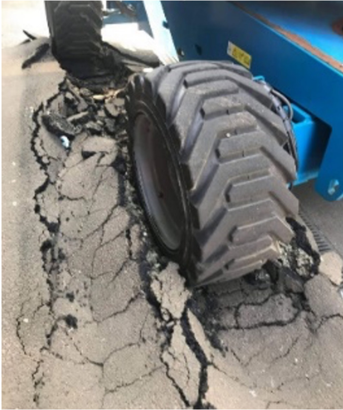
Example of ground sinking
