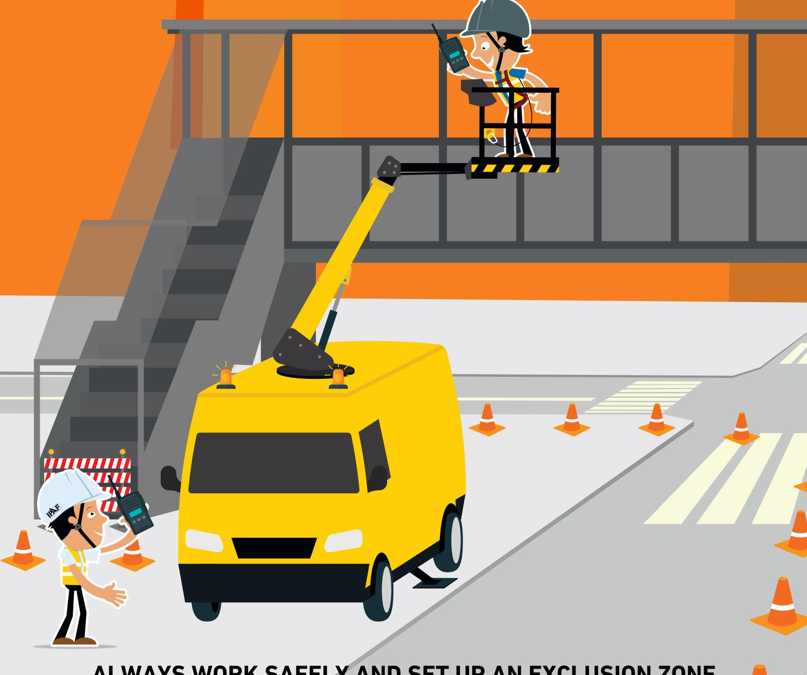
ALWAYS WORK SAFELY AND SET UP AN EXCLUSION ZONE TO PROTECT THE BOOM FROM ENTERING A LIVE ROAD
